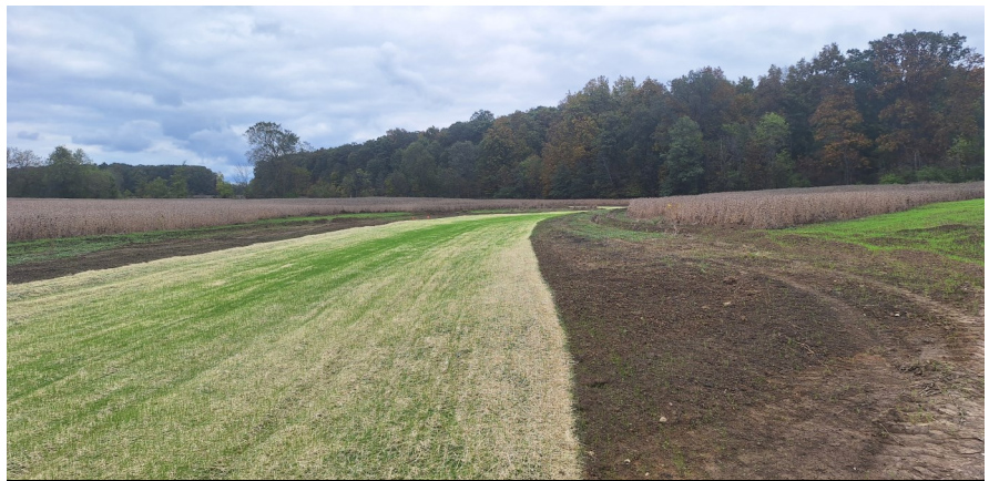
Newly installed waterway with mulch netting in place and grass growing.
