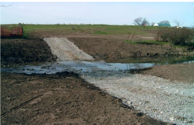
Recently installed low water crossing
